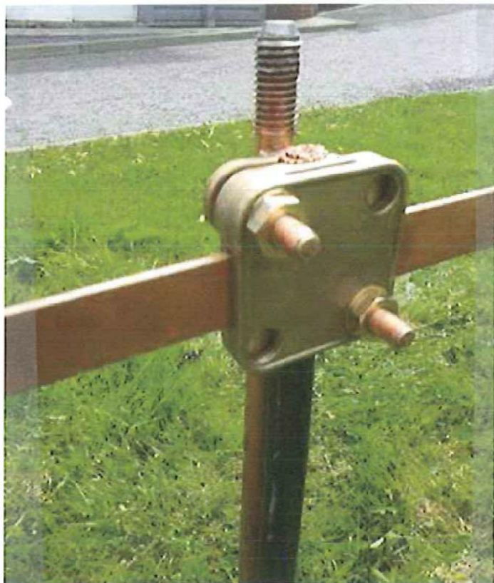
FIG. 1 – EARTH ROD CONNECTION POINT (Applies to all Sites)
