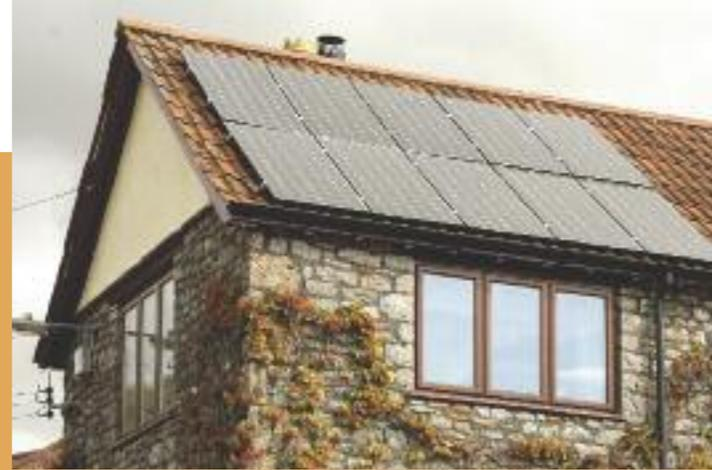
Solar panels are usually installed on south-facing roof surfaces in order to capture the maximum amount of sunlight available. The electrical conversion happens silently and without creating pollution.
