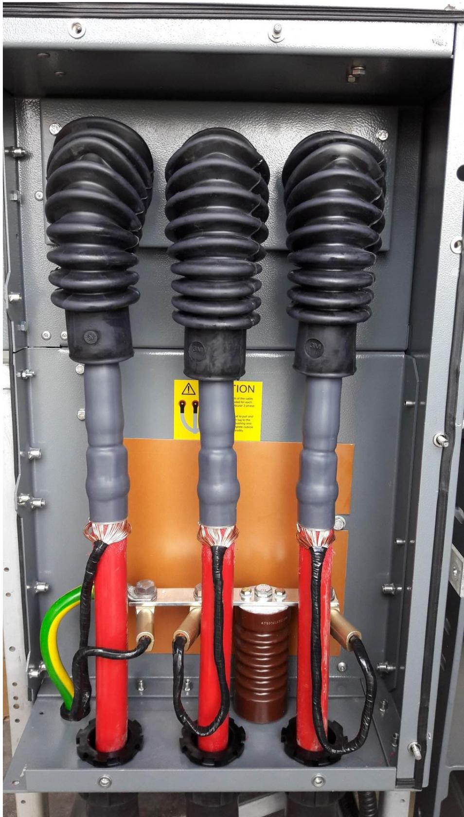
**3.20.9 Cable Sheath Earthing Arrangement**
