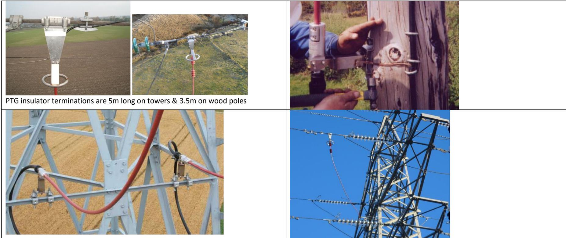
PTG insulator terminations are 5m long on towers & 3.5m on wood poles
